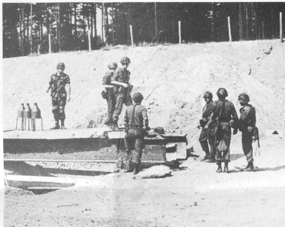
BLOWIN' IT—The 42nd Engineer Company spent time on the demoli-
